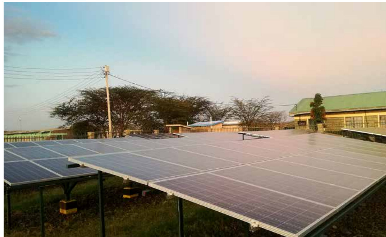
The 40kWp Solar Array that supplies the Solar PV hybrid mini-grid in Talek
