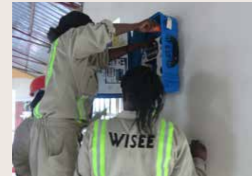
Installing a WSS solar suitcase at Tania Integrated Centre in Kiserian, Kajiado County
