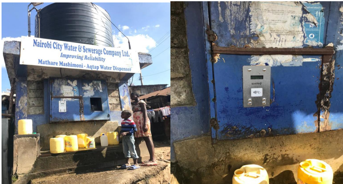
Fig 6&7: A water 'ATM' that is used to provide water for those with the transaction card in the Mathare area, Mwikali Racheal, 2020
