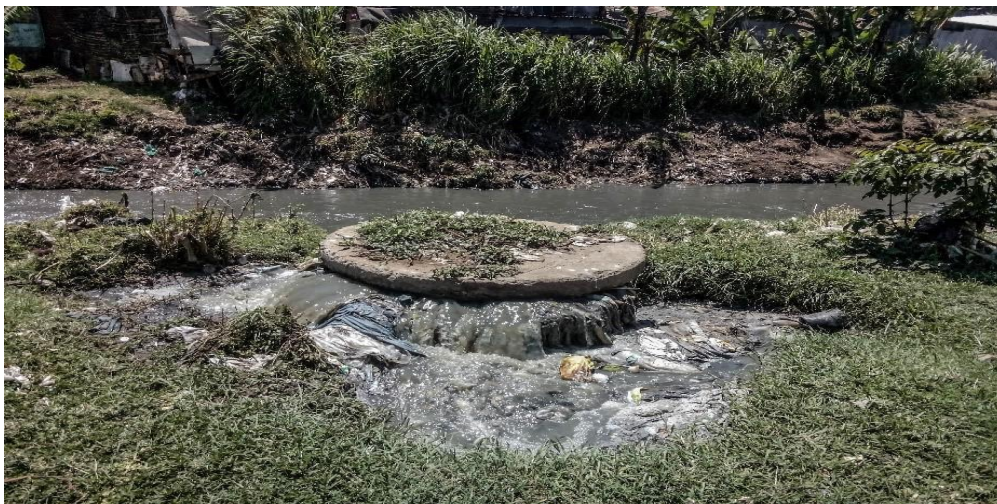
Fig 2: An overflowing sewage manhole, next to Nairobi River in Dandora. Alders Theodore, 2017
